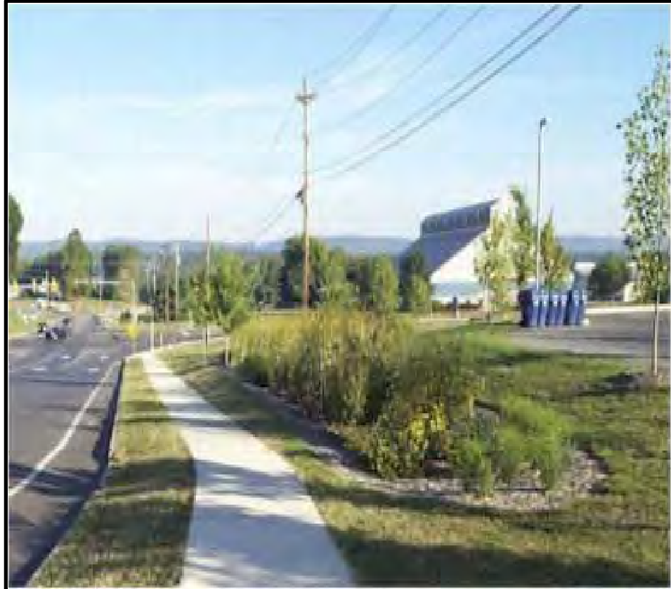
Photo 5-18. Pervious Concrete Along Roads and Streets
