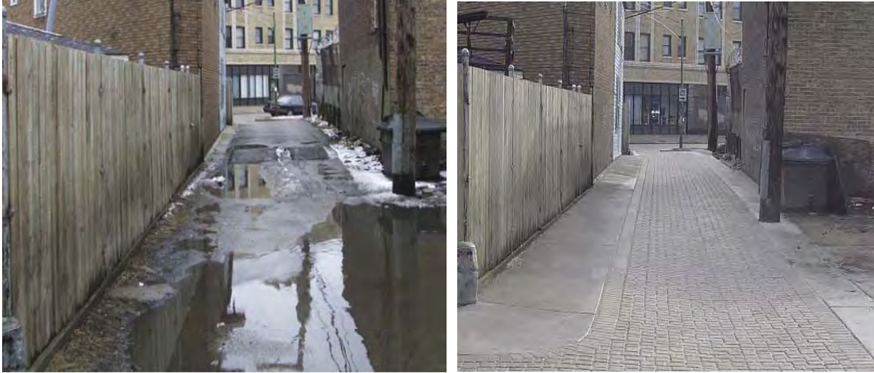
Photo 1-12: Before and After Drainage Improvement
