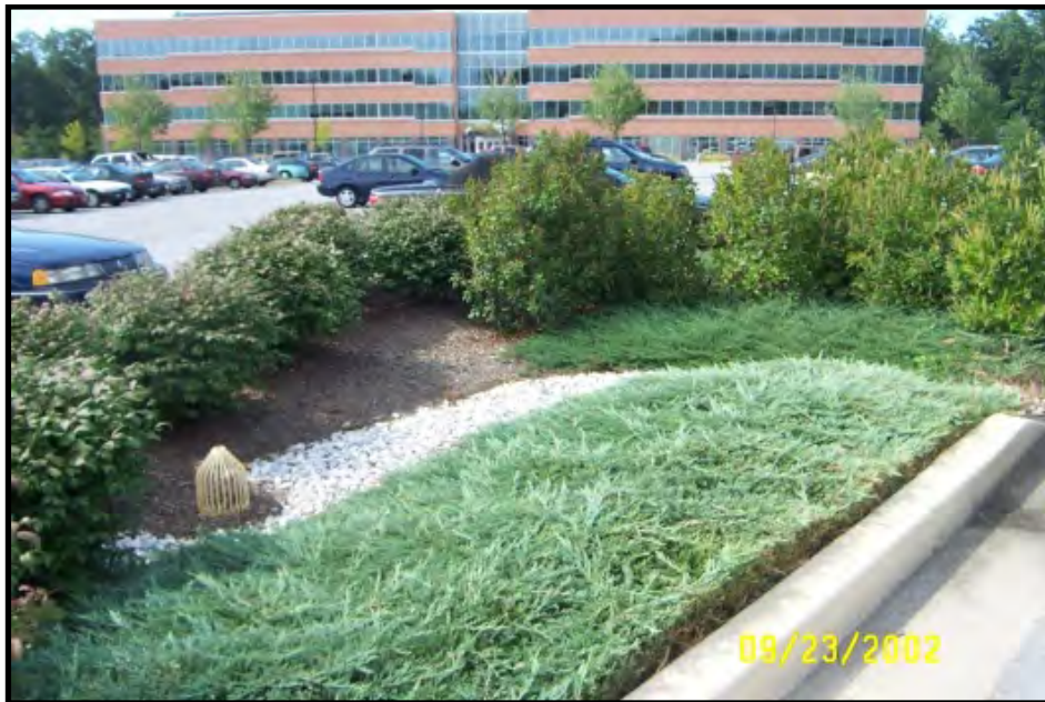
Photo 5-4. Inflow Entrance – Stone Channel
