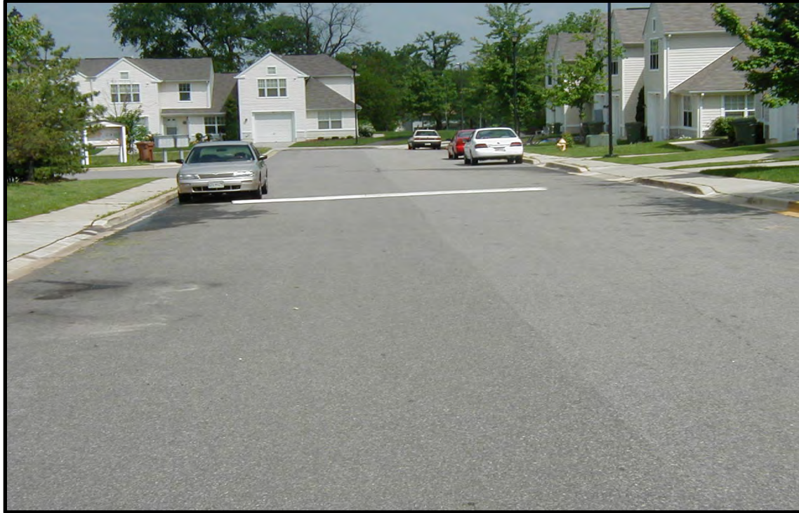
Photo 3-1. Typical Street for Military Housing (Source: UFC 3-210-10, 2004)
