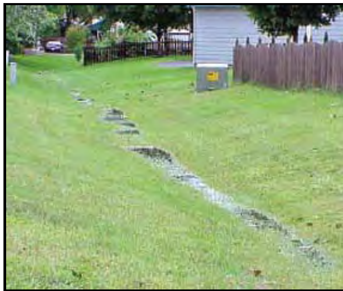
Photo 2-14. Grass Swale (Source: PA Stormwater IMP Manual, 2006)
