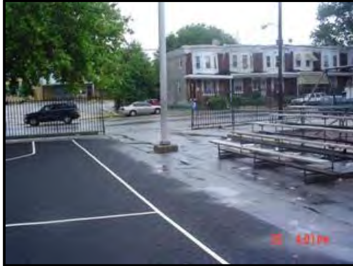
Photo 2-20. Pervious Pavement Basketball Court (Source: Philadelphia Water Department)
