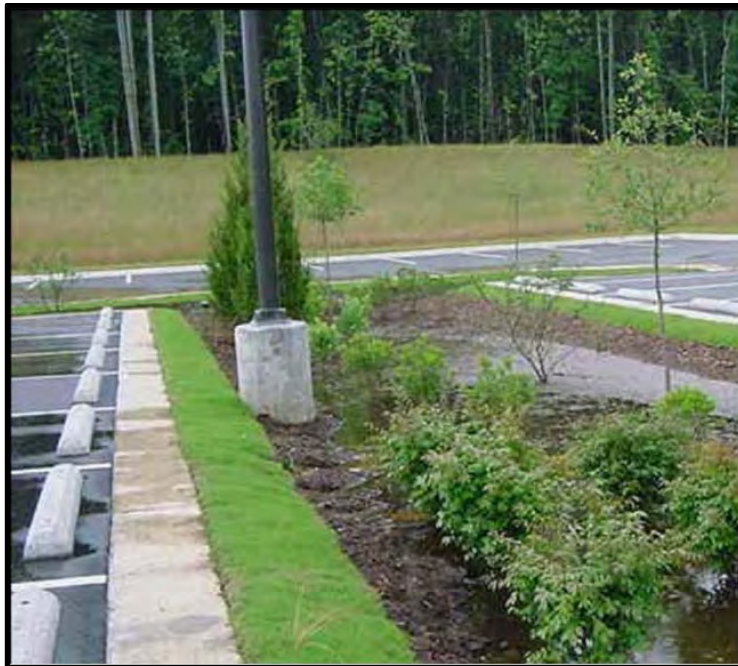
Photo 2-11. Bioretention (Source: USACE Savannah District)
