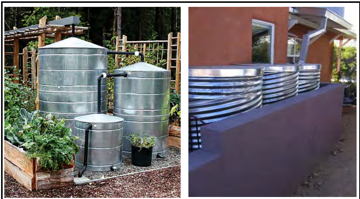
Photo 5-21. Linked Rainwater Harvesting Cisterns
