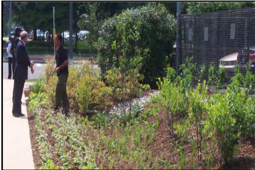
Photo 5-5. Mulch Layer in Bioretention
