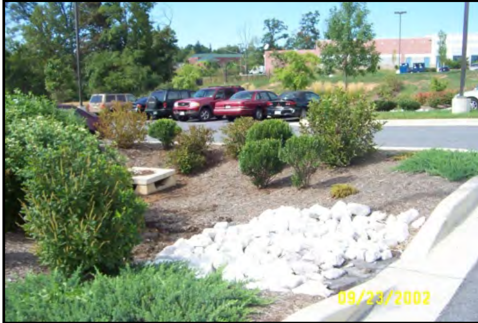
Photo 5-3. Inflow Entrance - Curb Cut with Riprap
