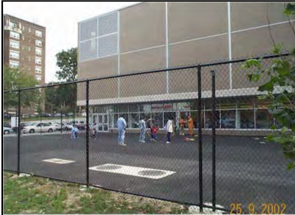
Photo 5-12. Porous Asphalt in Playground
