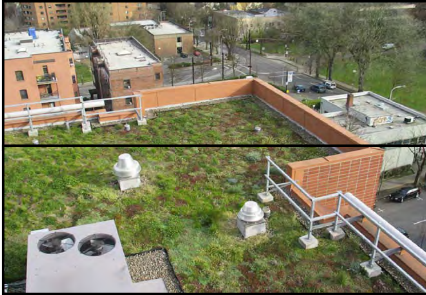
Photo 5-25. Hamilton Building Green Roof (Source: Portland Stormwater Management Manual)
