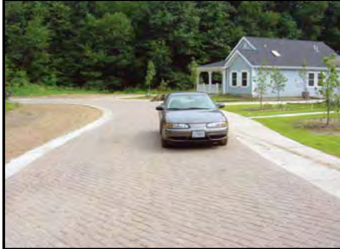
Photo 2-18. Permeable Concrete Pavers in Street in Dowagiac, MI (Source: Pokagon Band of Potawatomi Indians)
