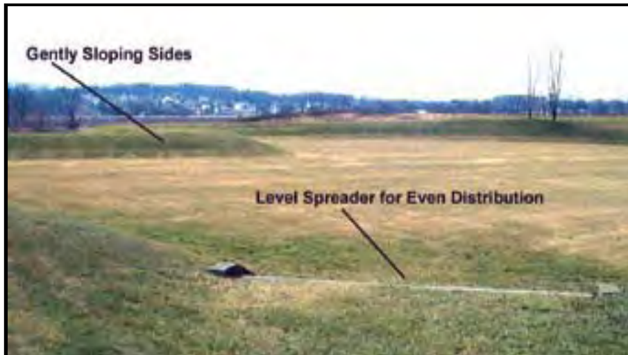
Photo 2-25. Infiltration Basin (Source: SEMCOG, 2008)
