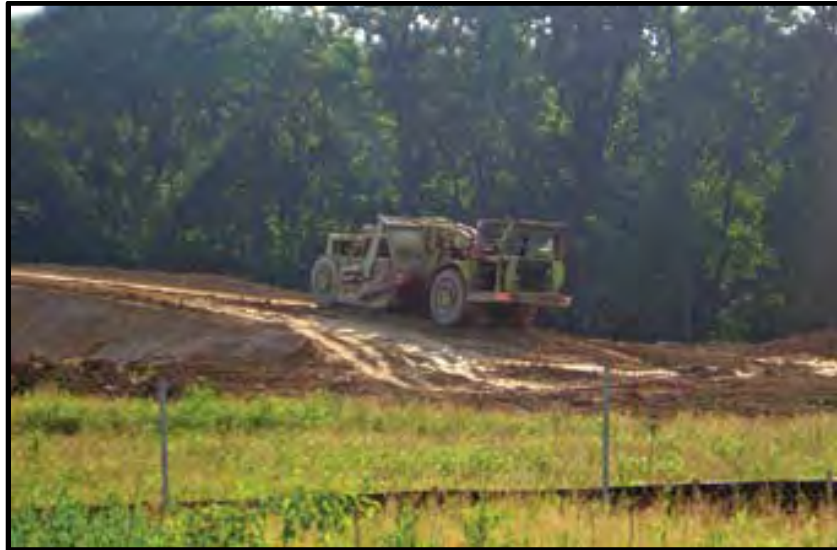
Photo 2-6. Construction Site Disturbance Showing Grading and Soil Compaction.
