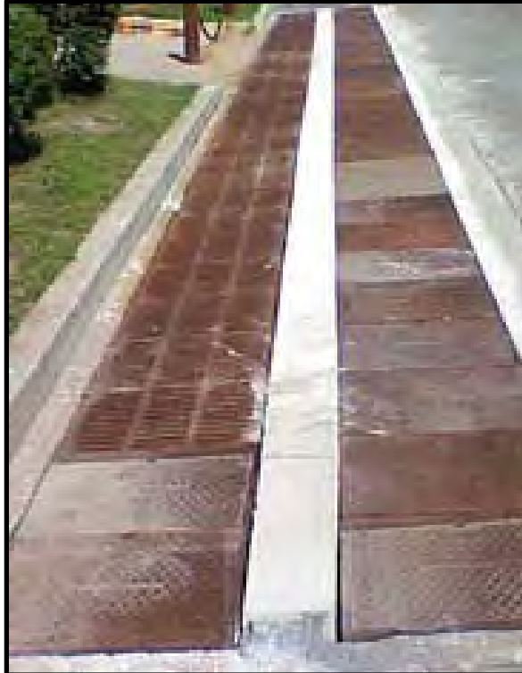
Photo 2-29. Two Chambered Sand Filter (Source: Wayne County, MI Department of Public Works)
