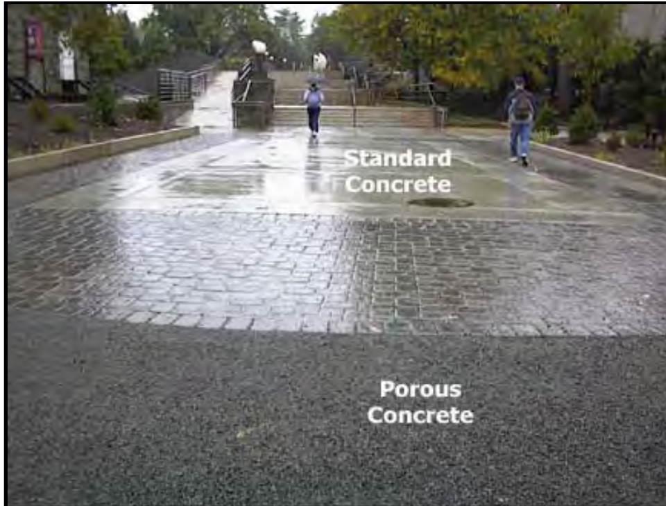
Photo 5-13. Standard and Porous Concrete
