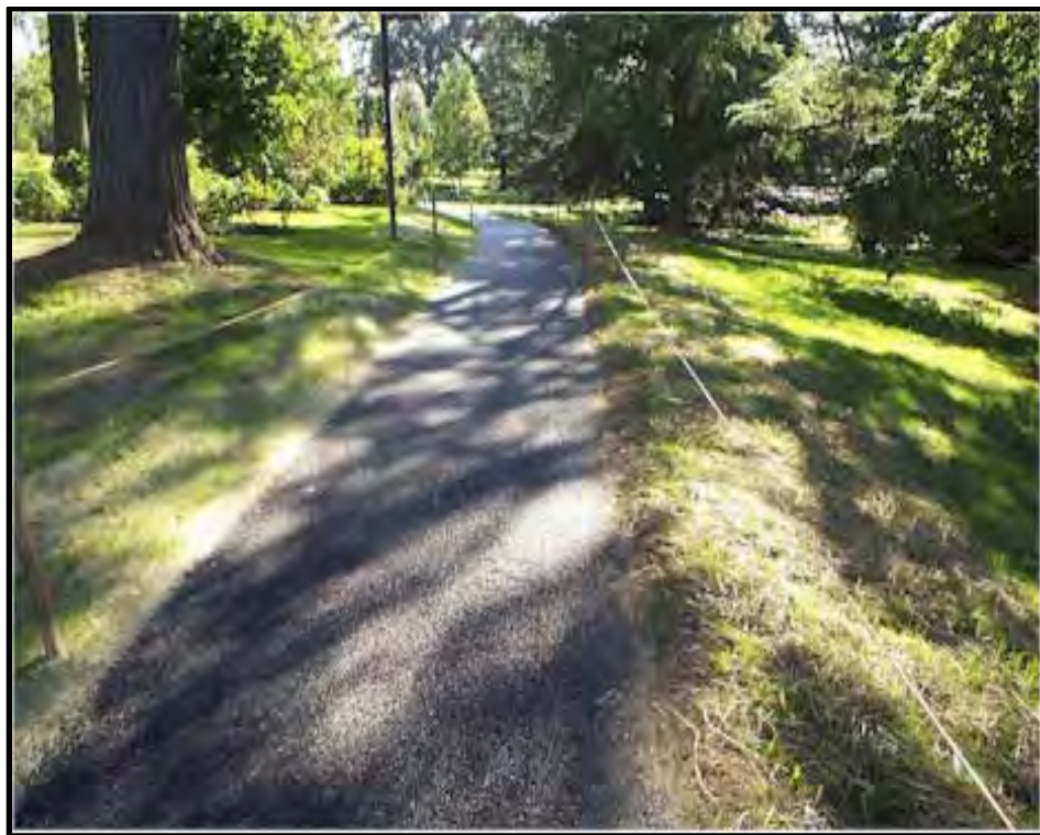
Photo 5-17. Porous Asphalt Along Pedestrian Walkways
