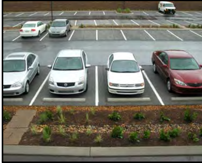
Photo 2-16. Permeable Pavement Parking Lot with Bioretention (Source: Hawkins Partners, Inc., 2009)
