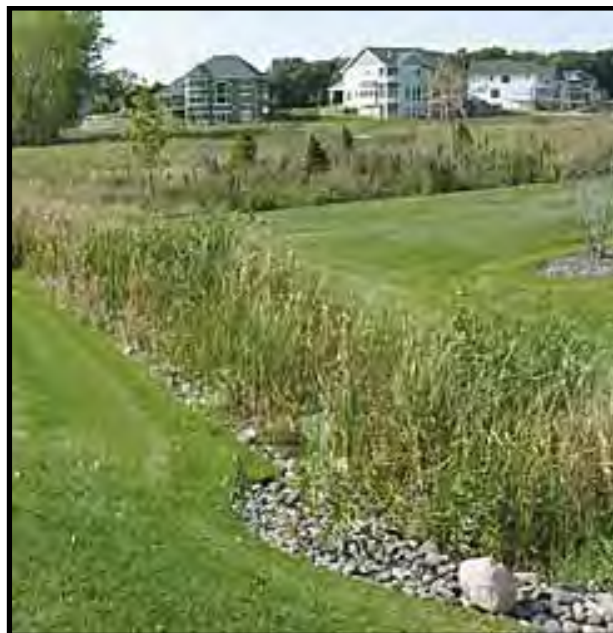
Photo 2-12. Vegetated Swale with Infiltration Trench (Source: USDA NRCS)
