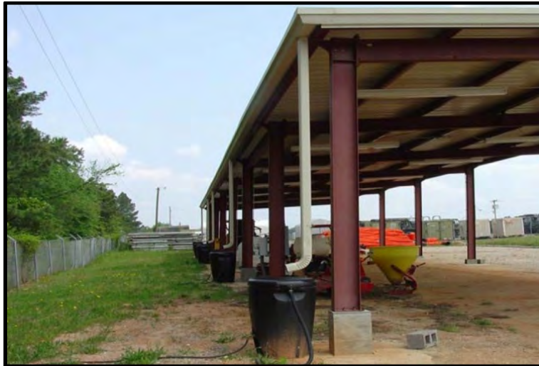
Photo 2-21. Rain Barrels for Rainwater Harvesting from Roof (Source: U.S. Army Fort Bragg)
