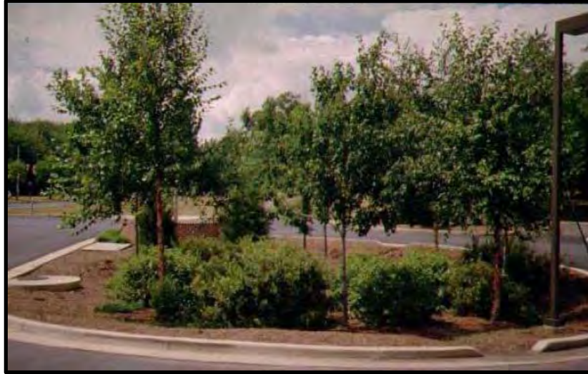
Photo 2-10. Bioretention in a Parking Lot (Source: Larry Coffman, 2008)
