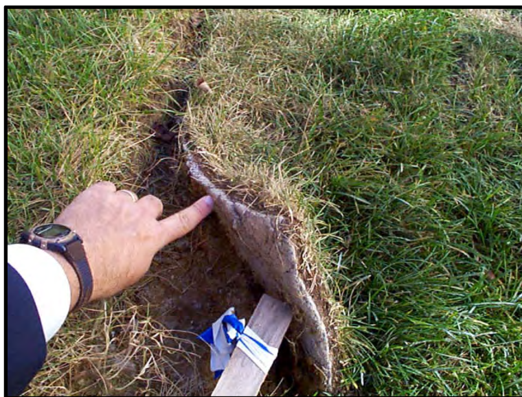
Photo 2-31. Compacted Soils (Source: Low Impact Development Center, Inc.)
