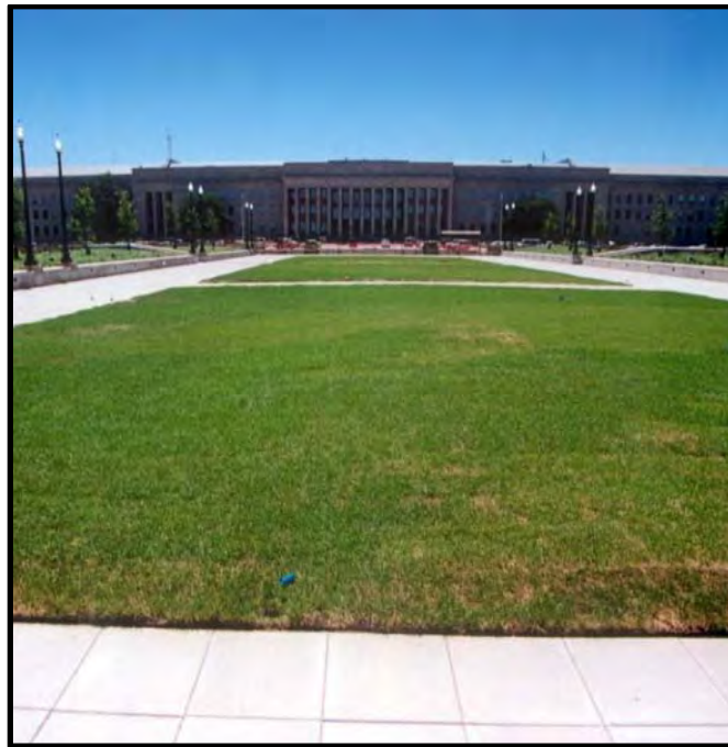
Photo 2-23. Green Roof at the Pentagon Remote Delivery Facility (Source: CAPT Robin Brake, 2008)
