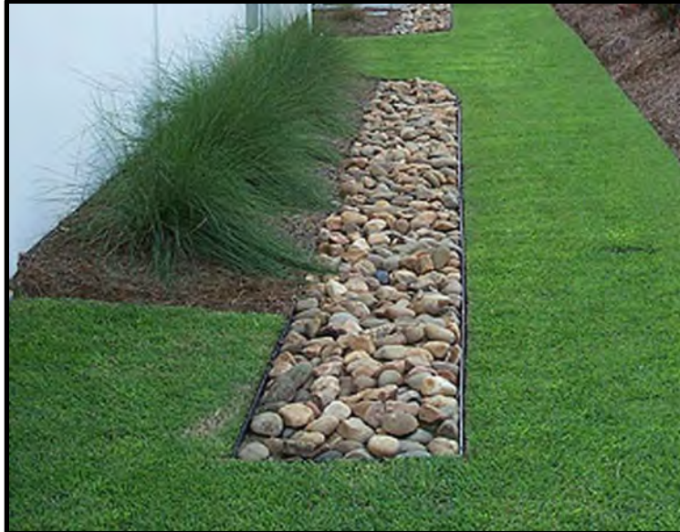
Photo 2-26. Infiltration Trench (Source: Tony Parker, Classic Landscapes, 2007)
