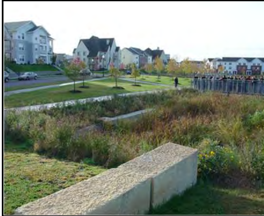
Photo 2-36. Treatment Train - Level Spreader and Vegetated Swale
