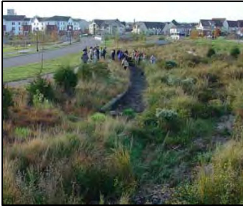
Photo 2-28. Level Spreader at the Edge of a Wetland Area
