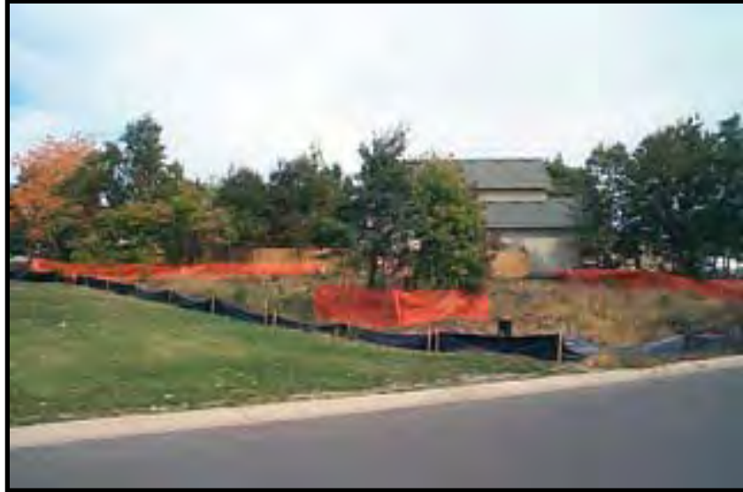
Photo 2-9. Protection of Vegetation on a Construction Site (Source: SEMCOG, 2008)
