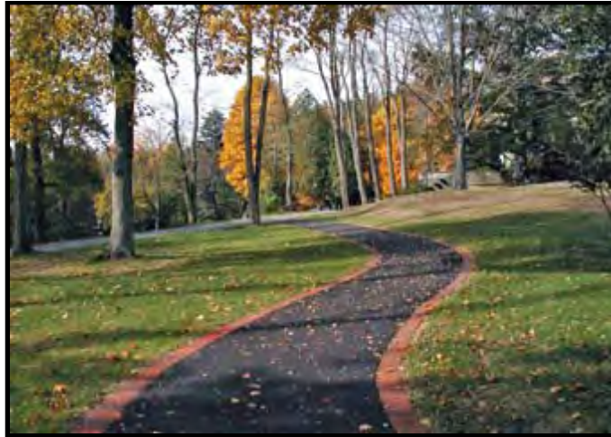
Photo 2-19: Porous Asphalt Pathway at Grey Towers National Historic Site, Milford PA (Source: SEMCOG, 2008)
