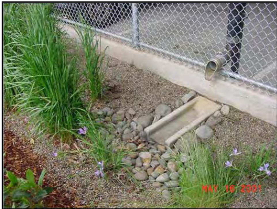
Photo 2-8. Downspout Disconnection to a Vegetated Area (Source: Prince George's County, MD Department of Environmental Resources)
