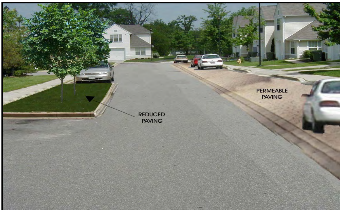
Photo 3-2. Street with Structural LID BMPs for Military Housing (Source: UFC 3-210-10, 2004)
