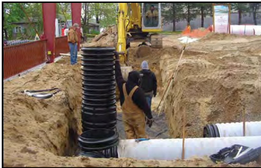
Photo 2-27. Installation of a Subsurface infiltration Bed (Source: Cardno JFNew)
