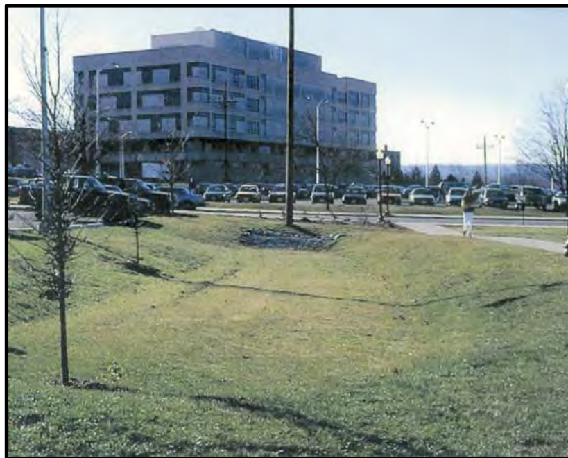
Photo 5-8. Vegetated Swale in a Commercial Setting
