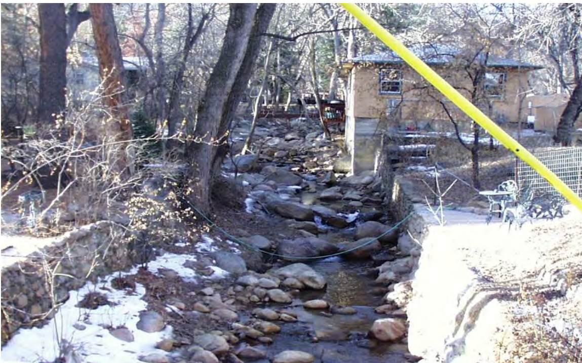
Photo 1-8. Floodplain encroachment on Cheyenne Creek in Colorado Springs.
