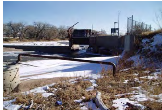
Photo 4-7. View of the gate at Clear Springs Diversion Dam.
