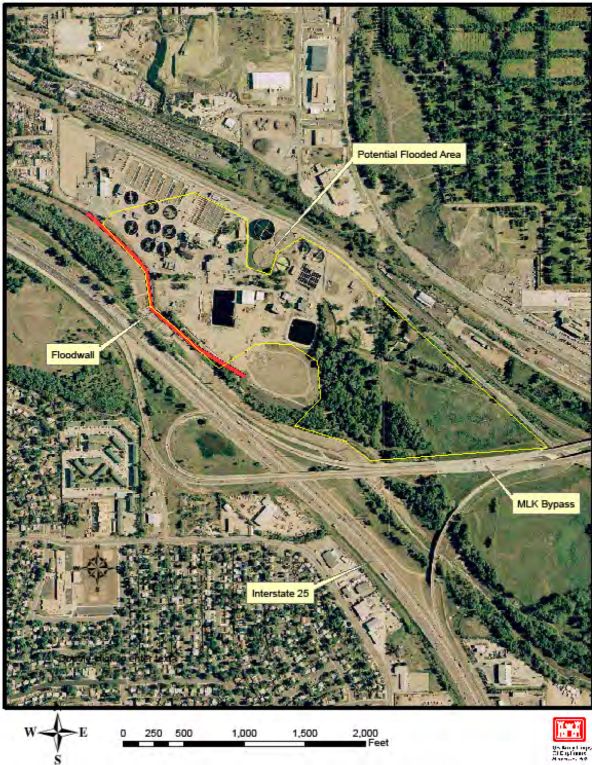
Figure 4-7. Flooding at Wastewater Treatment Plant.
