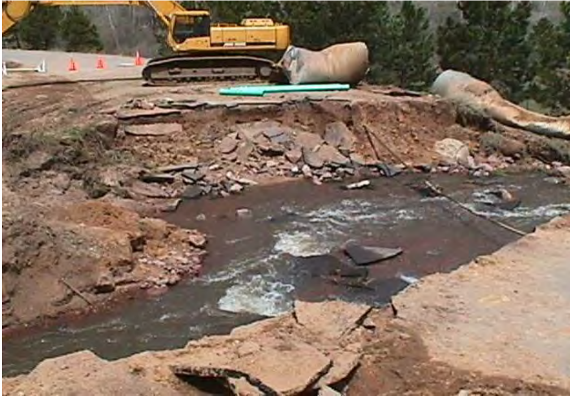
Photo 1-1. Flood damage in Palmer Lake.
