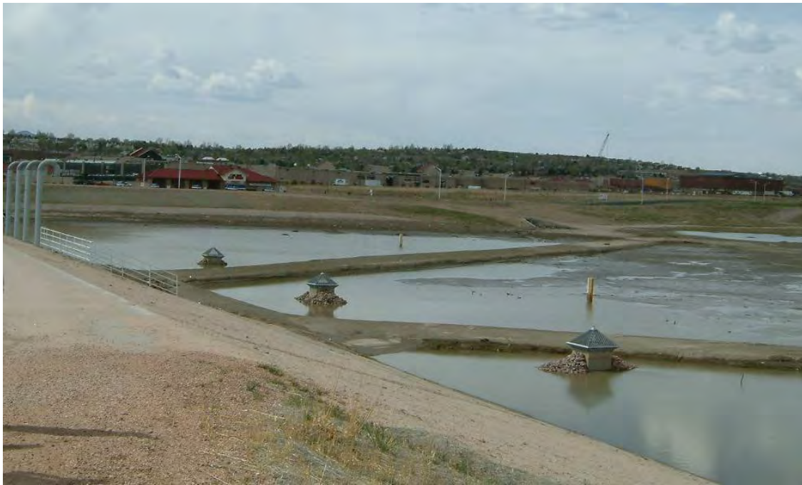
Photo 1-15. Sand Creek Detention Pond 1.
