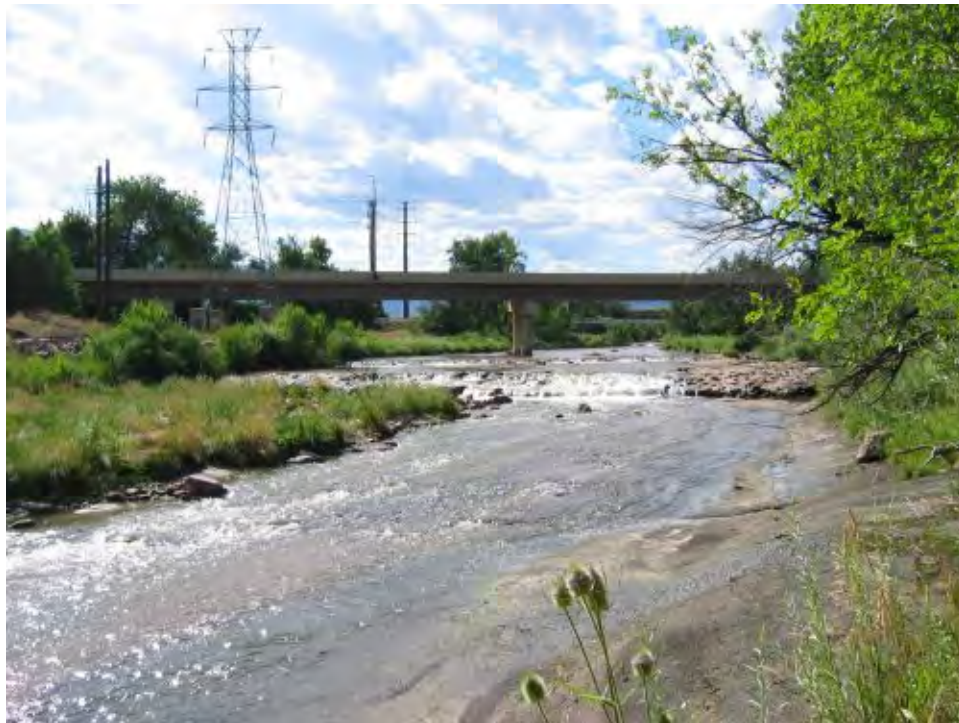
Photo 2-1. Fountain Creek below Martin Luther King Bypass/Hwy 24 Upstream view of double rock drop below on-ramp (0213)
