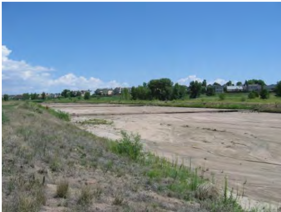
Photo 2-15. Sand Creek upstream of Constitution Avenue Upstream view of severely aggraded, channelized reach with drop structures (0281)
