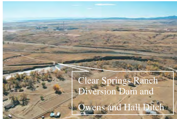
Photo 4-5. Aerial view of the Diversion Dam.
