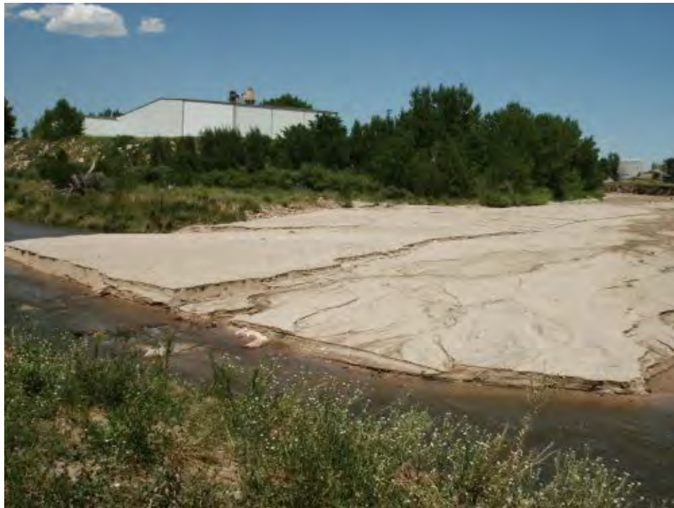
Photo 2-2. Fountain Creek at Sand Creek confluence Upstream view of Fountain Creek choked by Sand Creek sediment deposition (0003)
