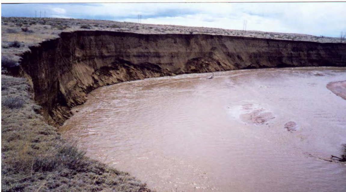
Photo 1-10. Erosion in El Paso County.
