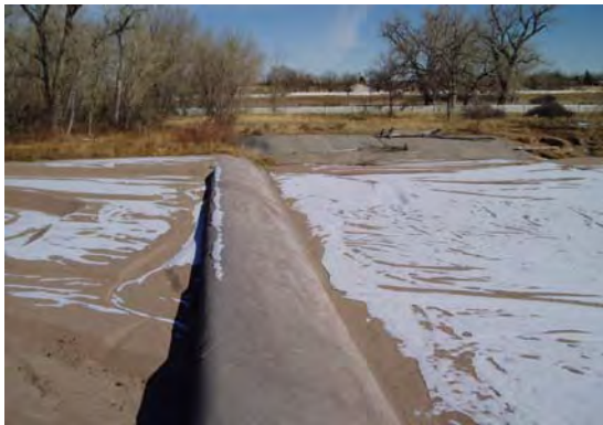
Photo 4-6. Drop structure at the dam.
