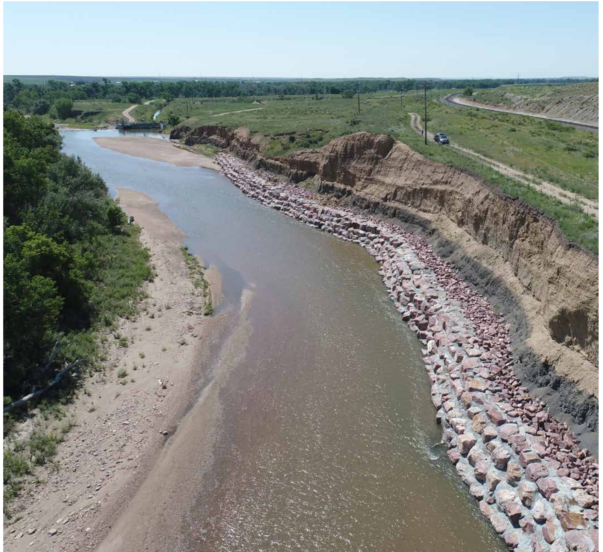
Bank Stabilization Fountain Creek
