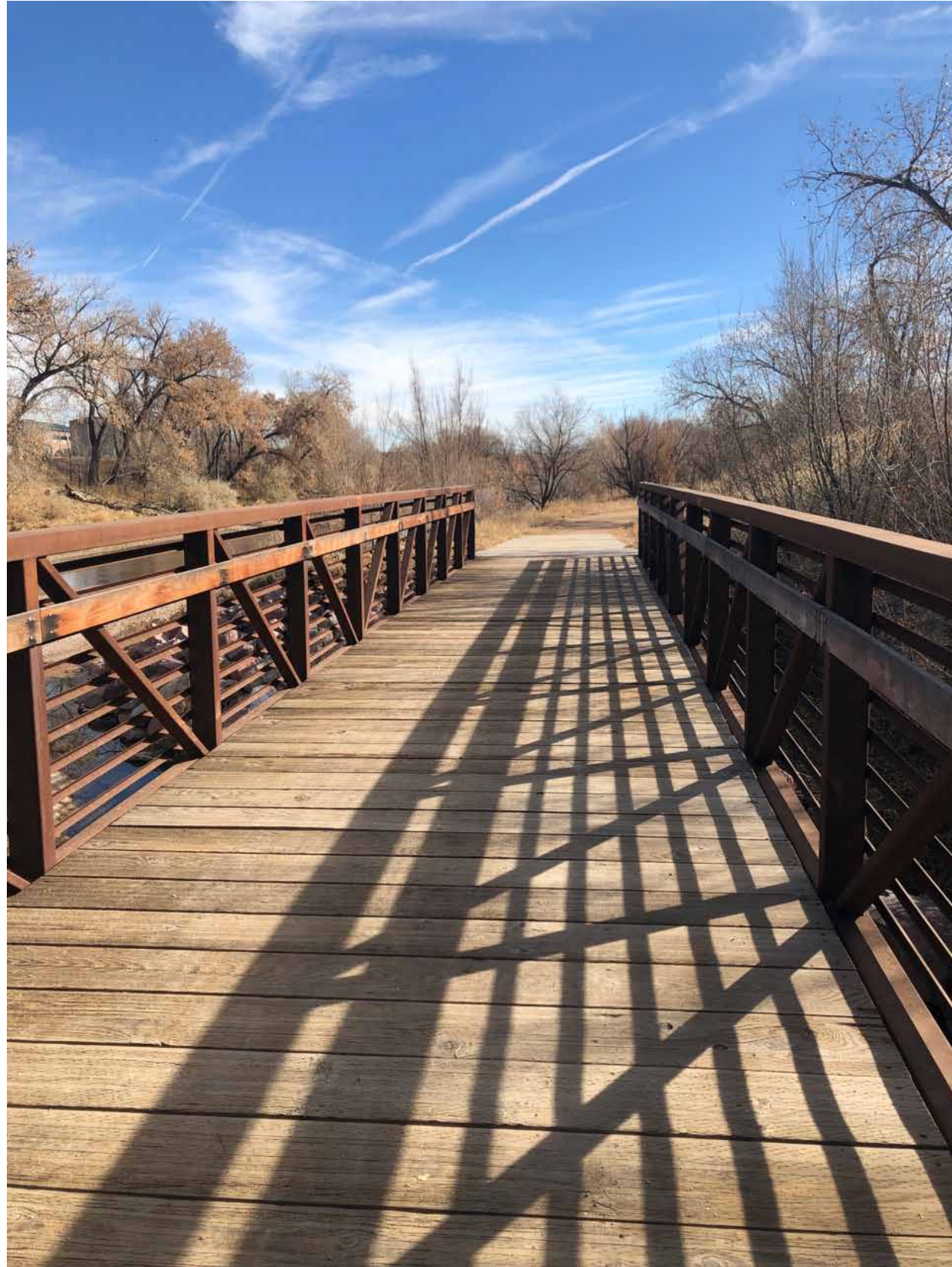
Pedestrian Bridge, Fountain Creek Greenway Trail
